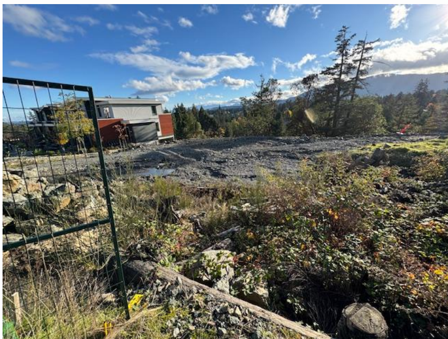
Views looking southwest from Manzanita Place to subject site. Bottom photo shows clearing that has taken place.
